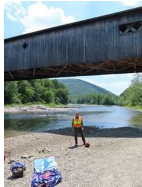
Ted at Dummerston Covered Bridge near Brattleboro, Vermont.
