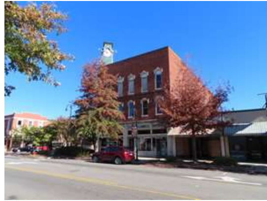
Building in Statesville, North Carolina.
