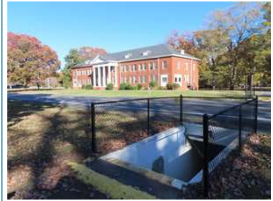
Building in Statesville, North Carolina.
