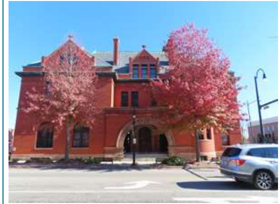
Building in Statesville, North Carolina.
