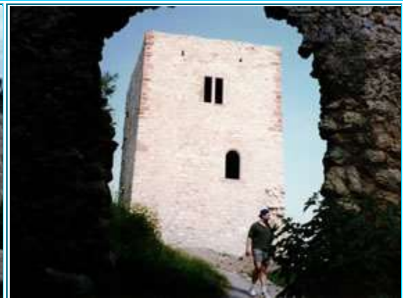
Two KM west of Eisenach Germany
