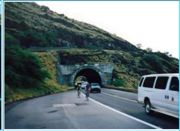
Other cyclists about to pass me after I went through a tunnel on highway 30 in Maui, Hawaii.
