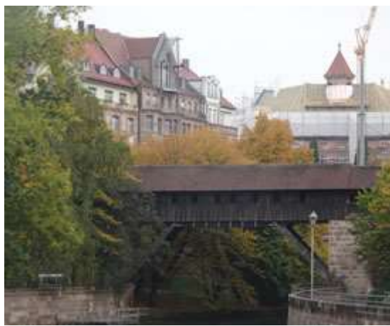
Covered bridge in Nuremberg, Germany.
